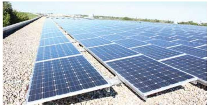
Powergate Plus 75 kW inverters, the resulting 367 kW array will generate almost 40% of United Displaycraft’s total estimated electricity needs – enough to power almost 50 average size homes in Illinois.
